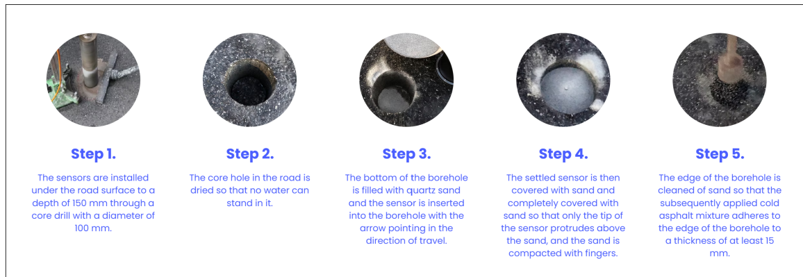
Figure 4: Installation process of traffic sensor magnetometers (CITIQ s.r.o, 2021)
